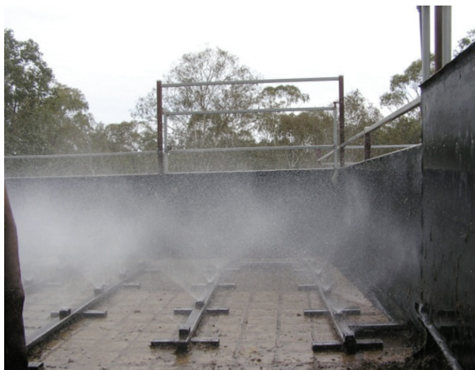
Photograph 1: Interior of a feedlot cattle wash showing ground mounted belly sprays
