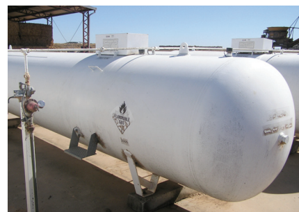
Figure 5: Gas meter installed beside the storage tanks
